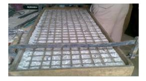
Fig.8: Strengthening slab by an additional ferrocement layer reinforced by GFRP mesh, SG
