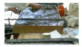
Fig.9: Casting concrete for strengthening layer
